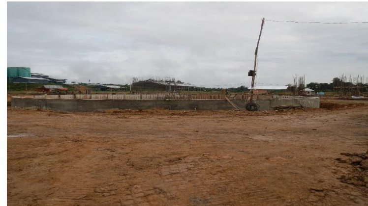
Reactor Tank Foundation
