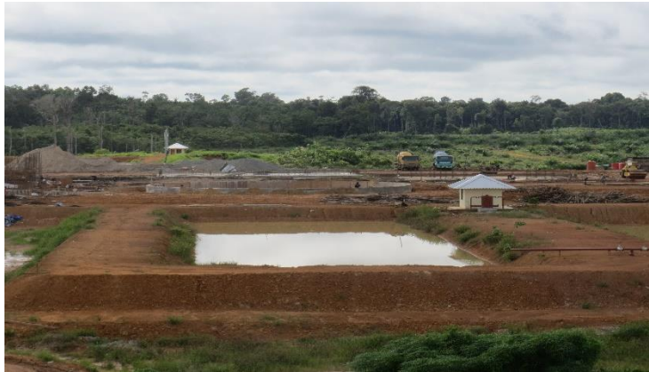
Cooling Ponds & Biogas Area
