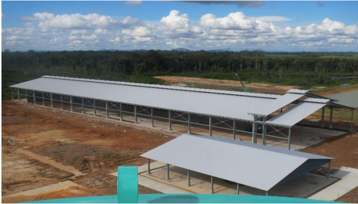
Bio-Compost Plant Area
